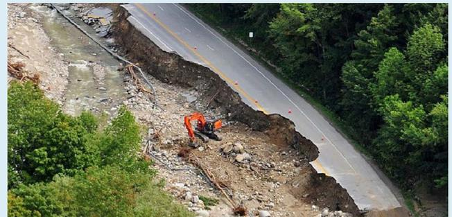
In 2011, Hurricane Irene caused major flooding and damaged infrastructure across Vermont, including this section of Route 107 in Stockbridge. Heavy storms are becoming more common as a result of climate change. Credit: Vermont Agency of Transportation.
